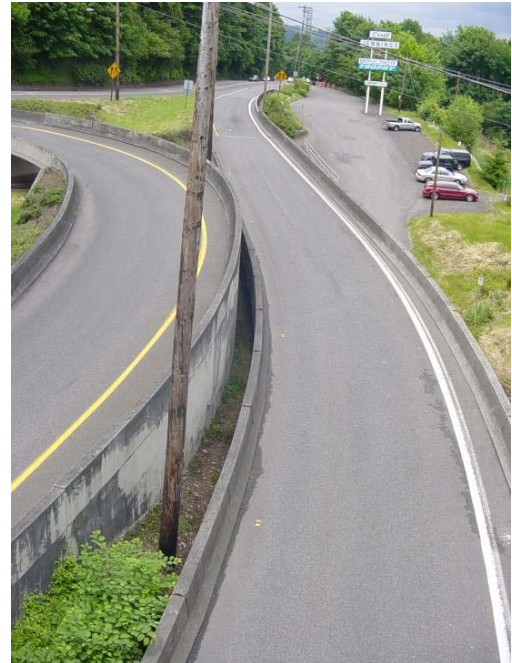
Figure 6: Northbound bypass ramp (to the right) as seen from the Sellwood Bridge.
