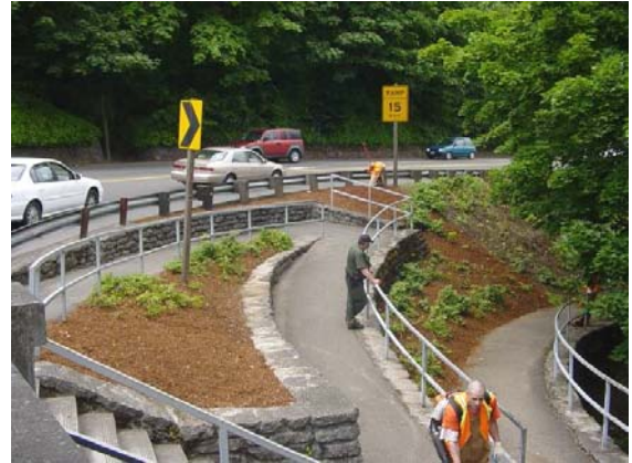
Figure 10: View of multi-use pathway, from Sellwood Bridge.
