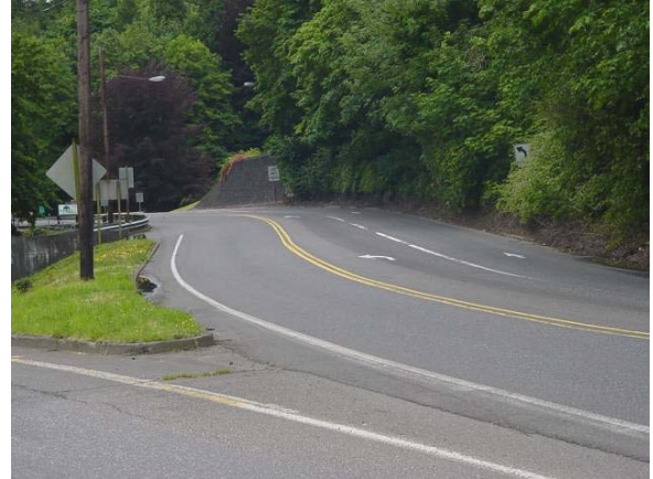
Figure 4: View of southbound left-turn lane from Highway 43 onto Sellwood Bridge.
