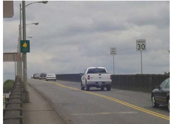
Figure 9: Looking eastward onto the Sellwood Bridge.
