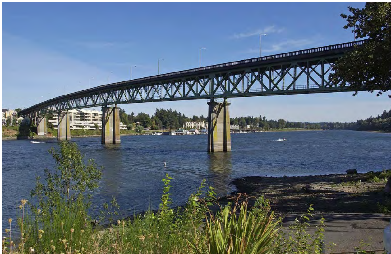
The existing Sellwood Bridge.
