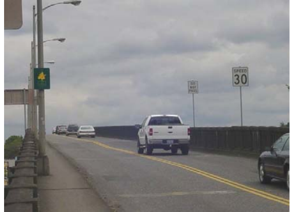
Figure 9: Looking eastward onto the Sellwood Bridge.
