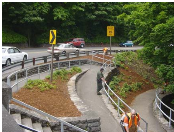
Figure 10: View of multi-use pathway, from Sellwood Bridge.
