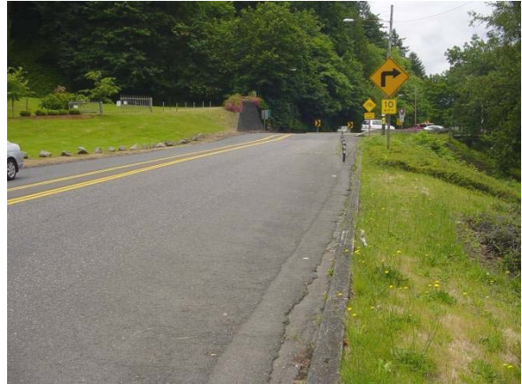
Figure 5: No sidewalks, crosswalks, or bicycle lanes exist on the mainline of Highway 43 in the vicinity of the Sellwood Bridge.
