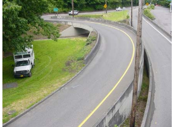
Figure 7: Southbound loop ramp (to left) as seen from Sellwood Bridge.
